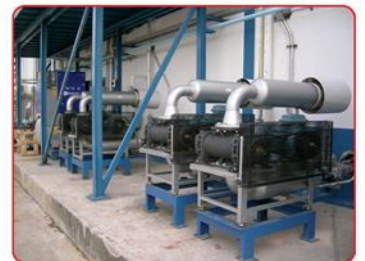
Roots Blower Installation
