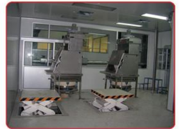
Manual Dump Station, Food Industries
