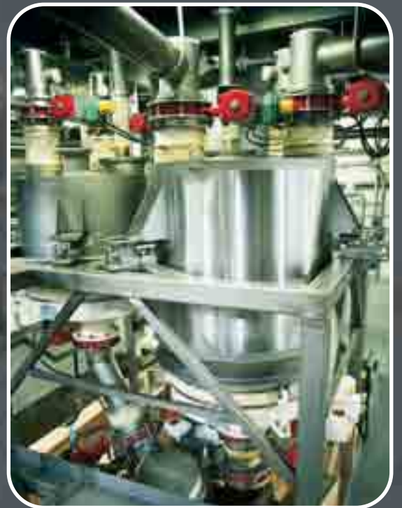
SANITARY BATCH PLANT INSTALLATION
