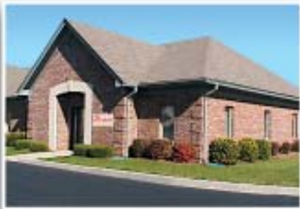
Regional Office, Avon (Indianapolis), Indiana
